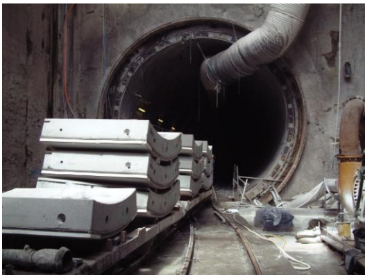
TBM Construction Box Interface
